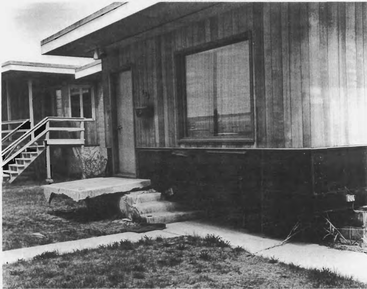
29.—House pushed off foundation by pressure ridge at toe of L Street slide. Well-framed house not otherwise visibly damaged. Push must have been shallow and nearly horizontal.
