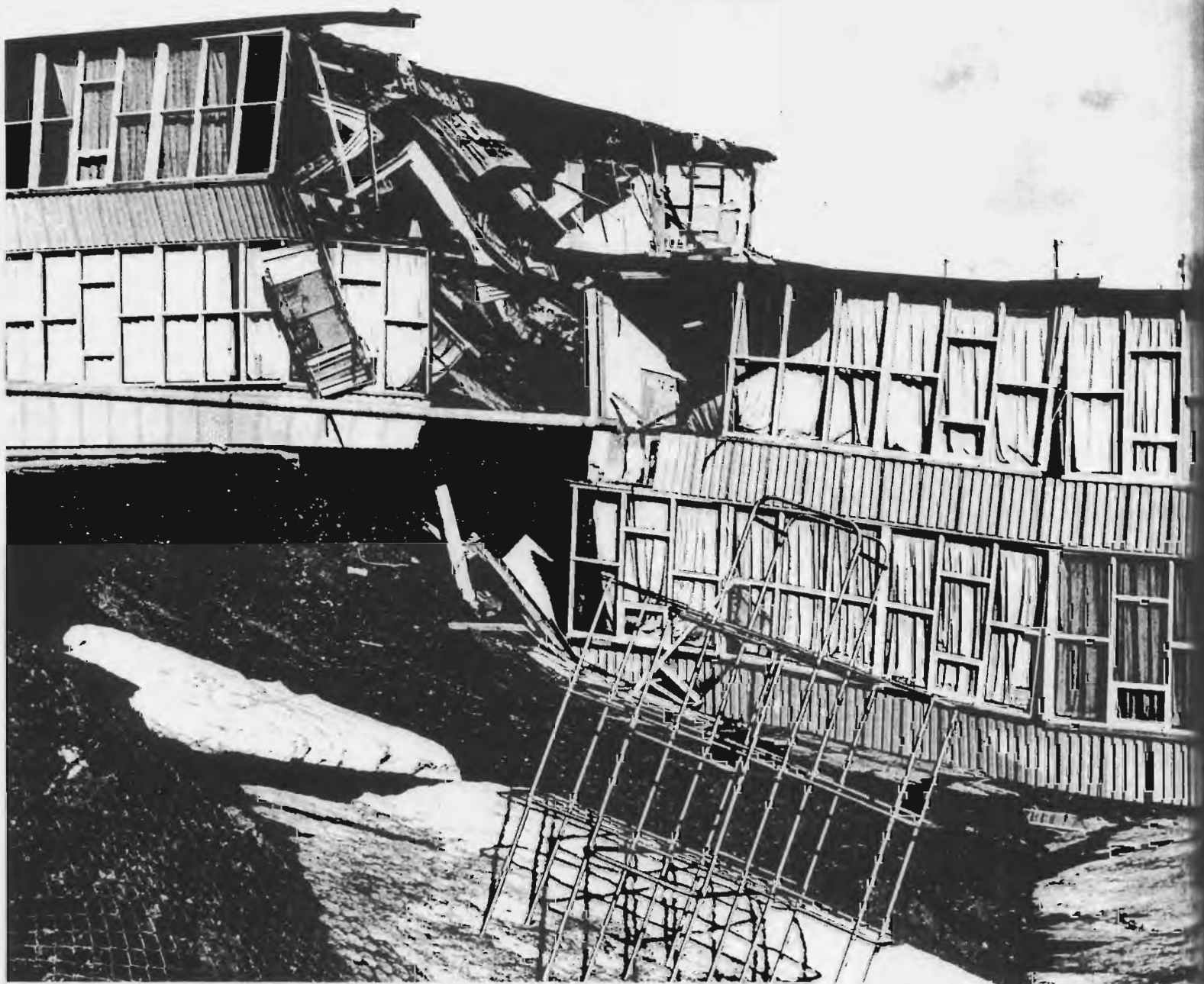
3.—Wreckage of Government Hill School. The south wing of the building, shown here, collapsed into a graben at the
