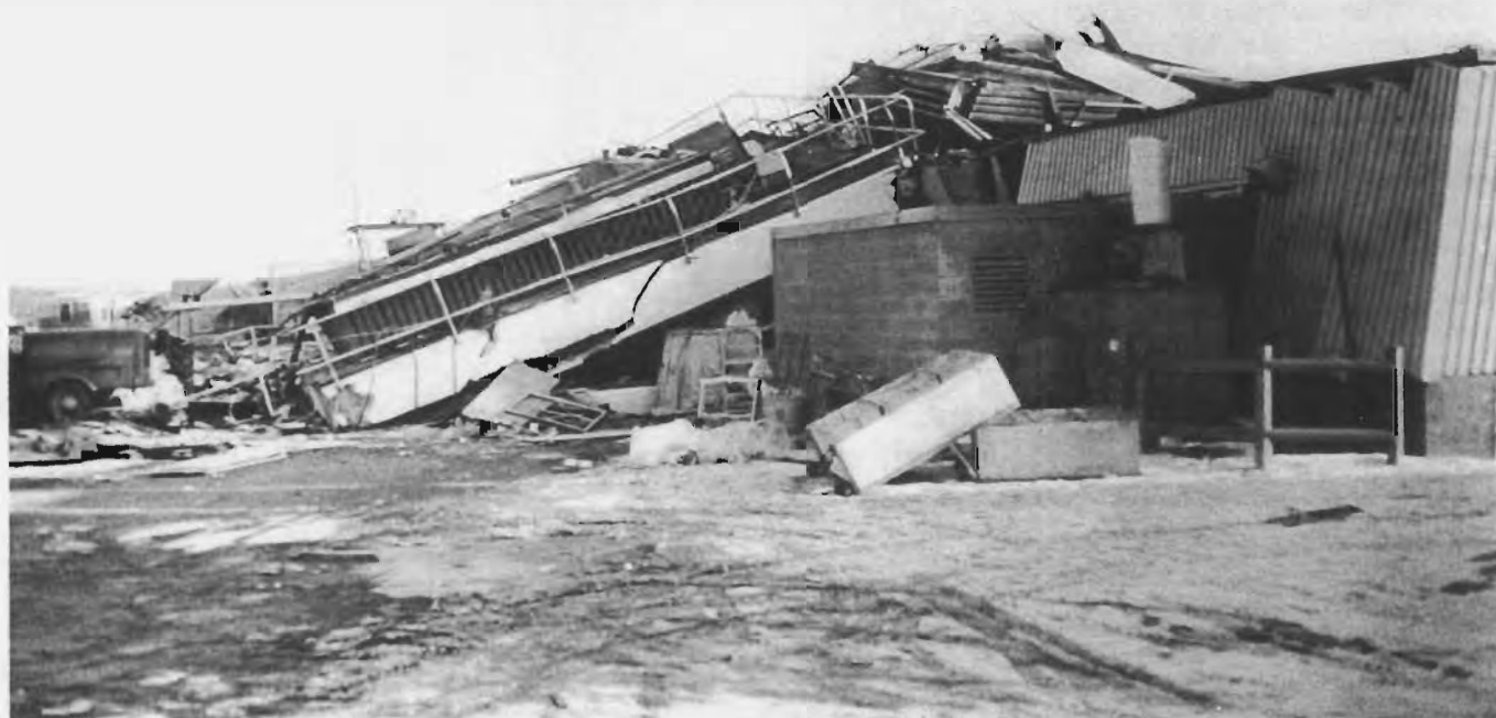
7.—Wreckage of control tower at Anchorage International Airport. Six-story tower failed under sustained seismic shaking. Photograph by George Plafker.
