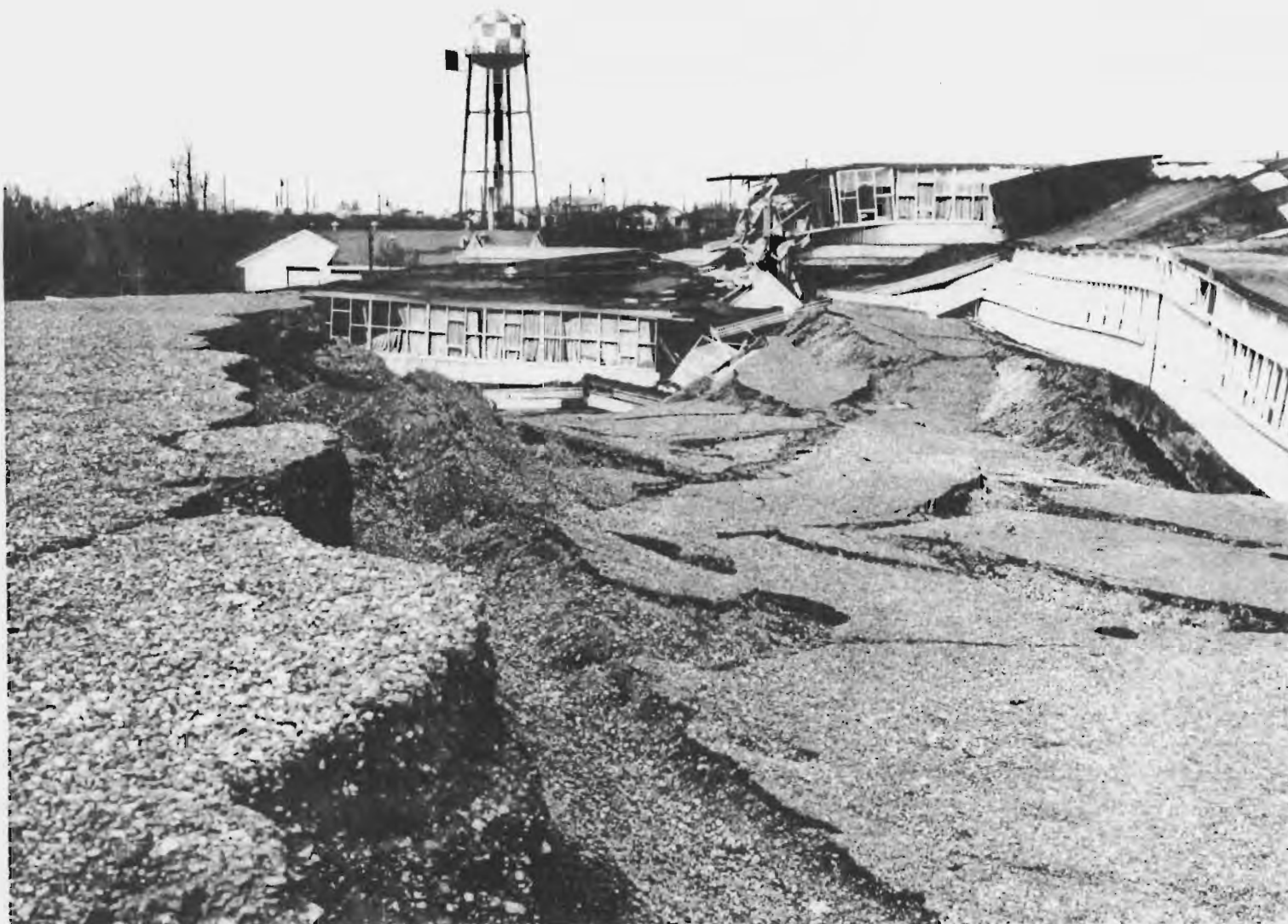
36.—Wreckage of Government Hill School as viewed from the playground, looking west. Graben in foreground is about 12 feet deep. Note undamaged water tower.
