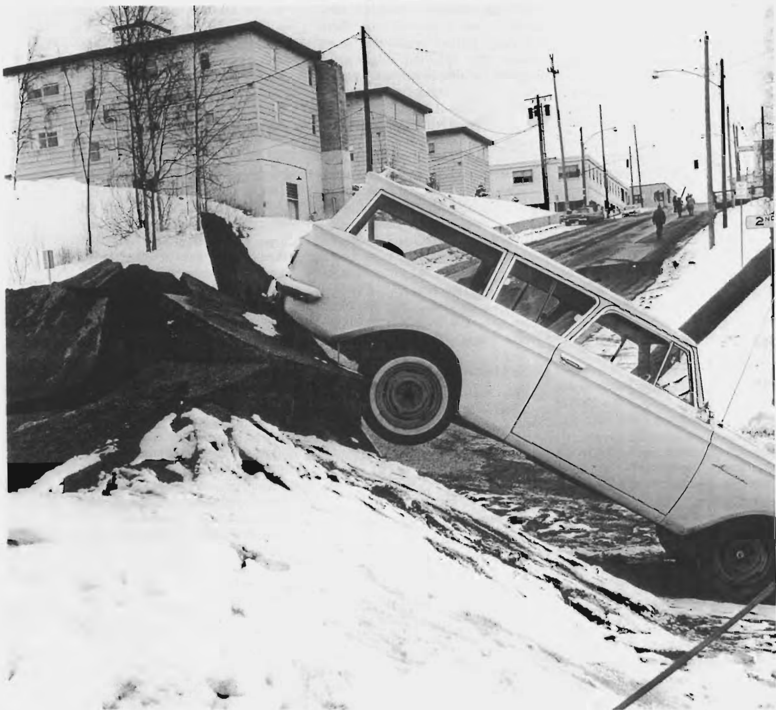
26.—Sharp-crested pressure ridge at Second Avenue and C Street, Anchorage. Probably caused by shallow translation of frozen surface layer. Note smaller pressure ridge in street part way up block and toppled chimney of building behind car. Photograph by Mac's Foto, Anchorage.
