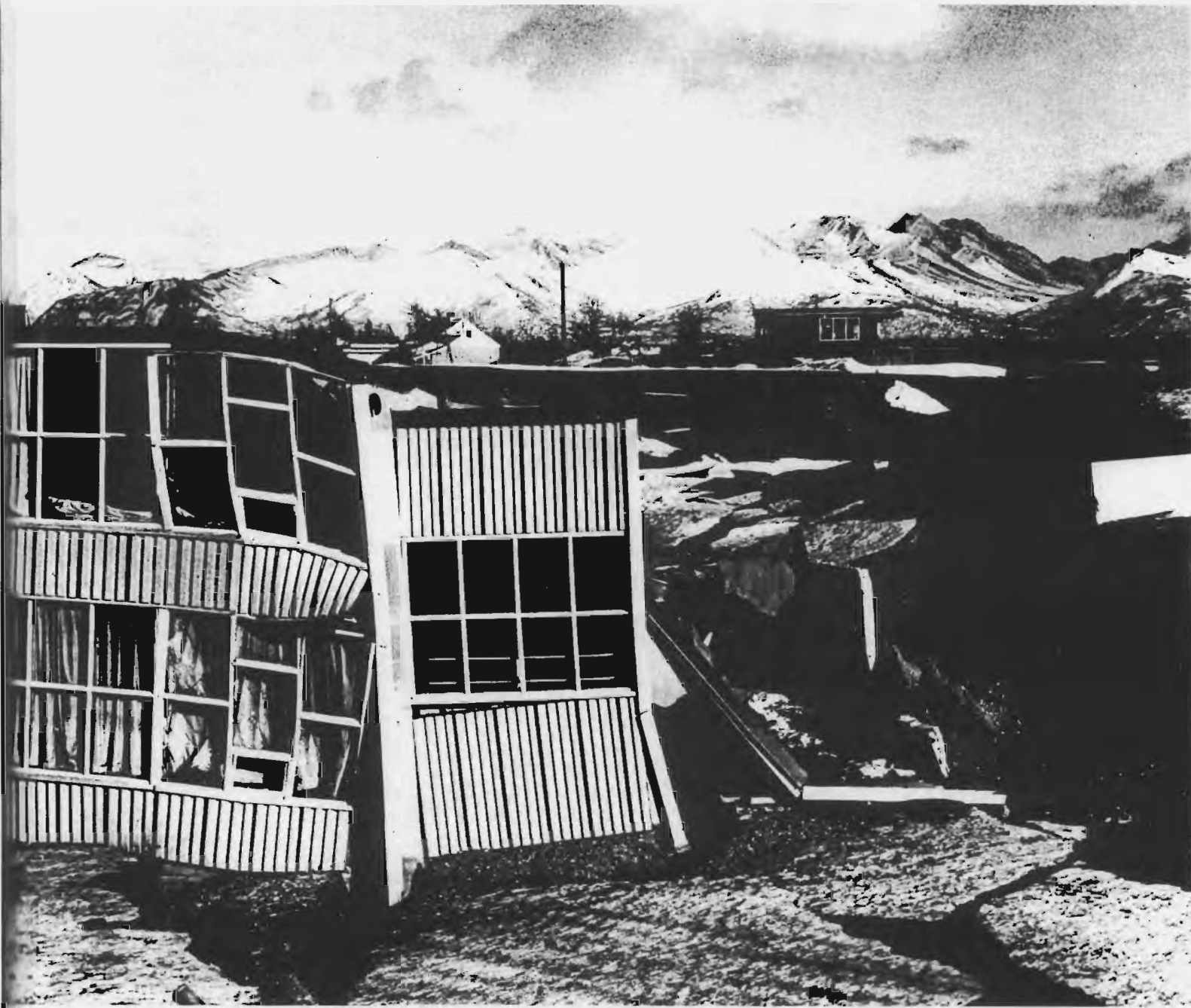
head of the slide. Net slip of the graben block is shown by the displacement of the roofline. Photograph by M. G. Bonilla.
