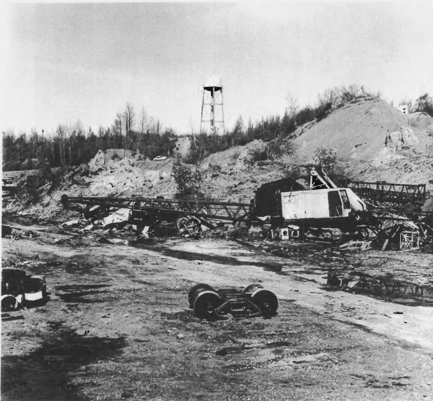
6.—Damage to yards of The Alaska Railroad, looking northwest, caused by earthflow at toe of Government Hill slide. Note undamaged water tank in background.
