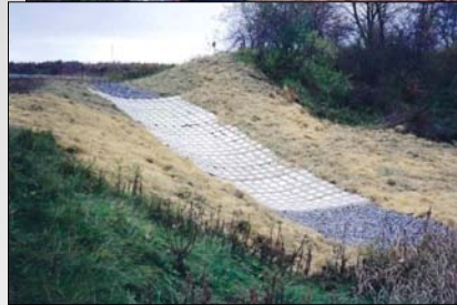
East Slope Erosion Controls
