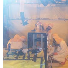
Size-reducing a glove box in the Container Size Reduction Facility
