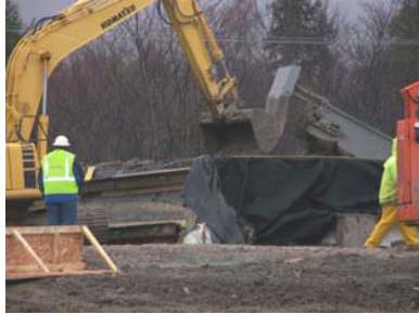
Permeable Treatment Wall installation
