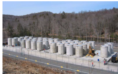
The completed WV storage pad will look similar to the one pictured above.
