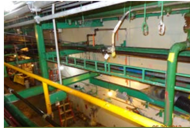
Interference Piping Removal in COA
