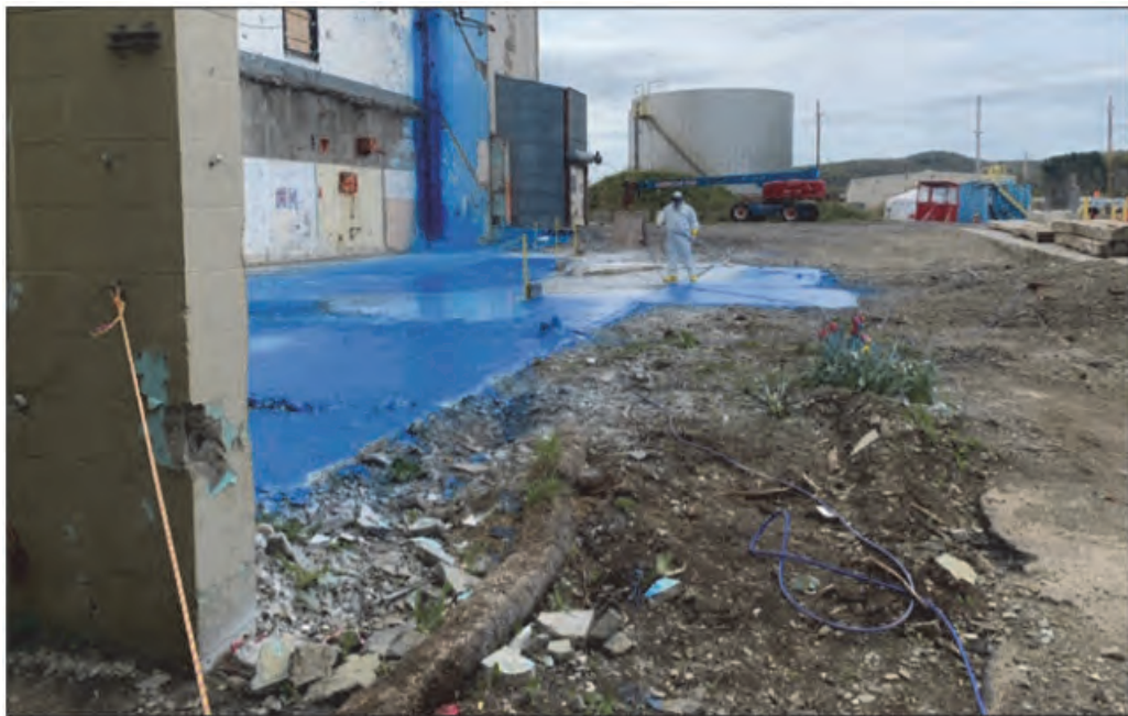
A worker at the West Valley Demonstration Project applies Polymeric Barrier System (PBS) to the concrete slab of the former main plant office building.
