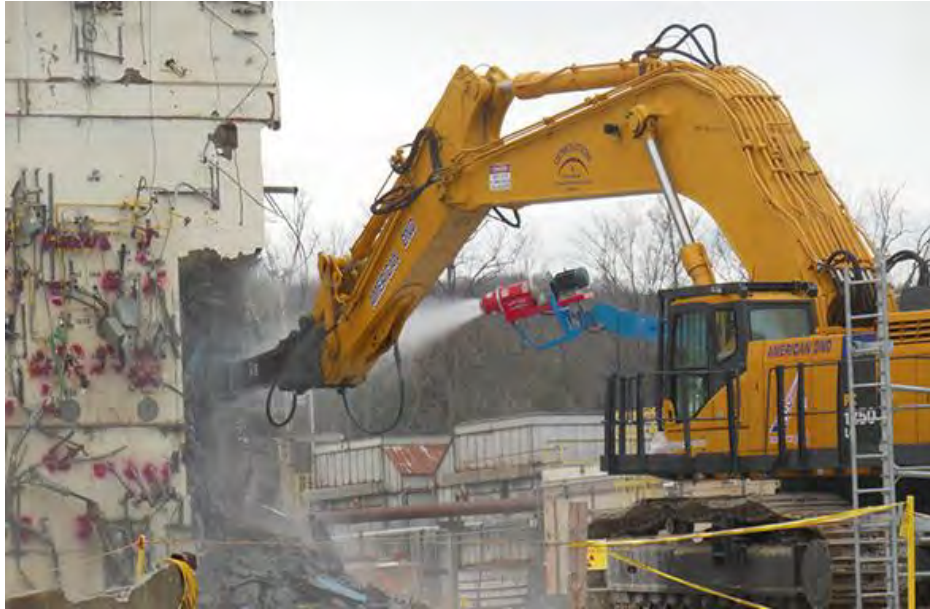
Crews take the “first bite” of the Vitrification Facility during the second phase of demolition.
