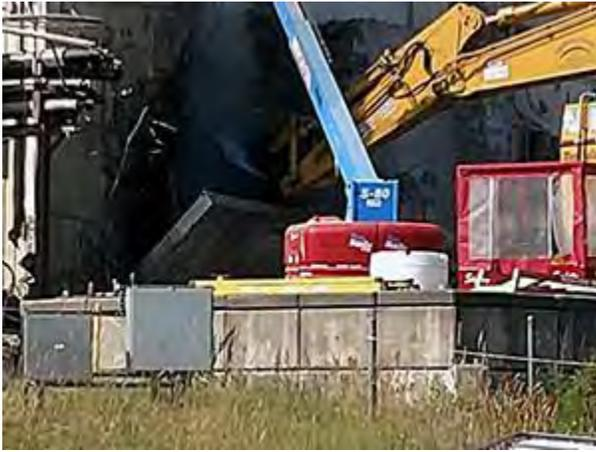
*Heavy equipment lowers the 60-ton transfer tunnel shield door to the ground.*
