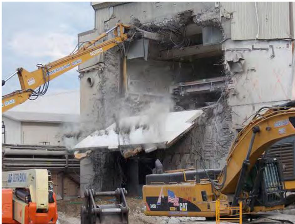
*Crews use equipment to loosen and lower the 100-ton crane maintenance room shield door from the Vitrification Facility.*
