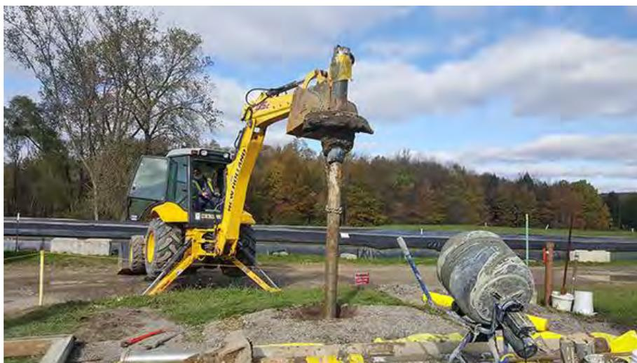
*A backhoe is used to pull the well pump and casing from the ground after workers stabilized the casing with grout.*
