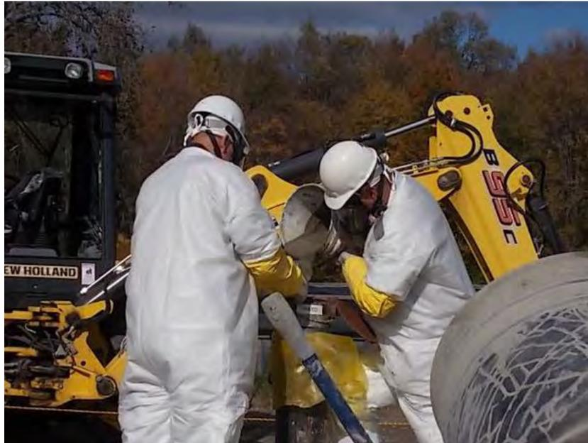
*Crews pour grout into the well pump casing to stabilize it before pulling out the well pump.*
