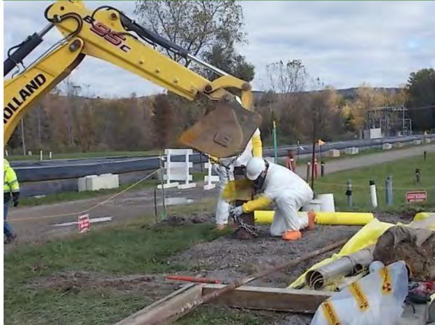
*Workers prepare to remove a well pump from a former pump-and-treat system at EM's West Valley Demonstration Project site.*
