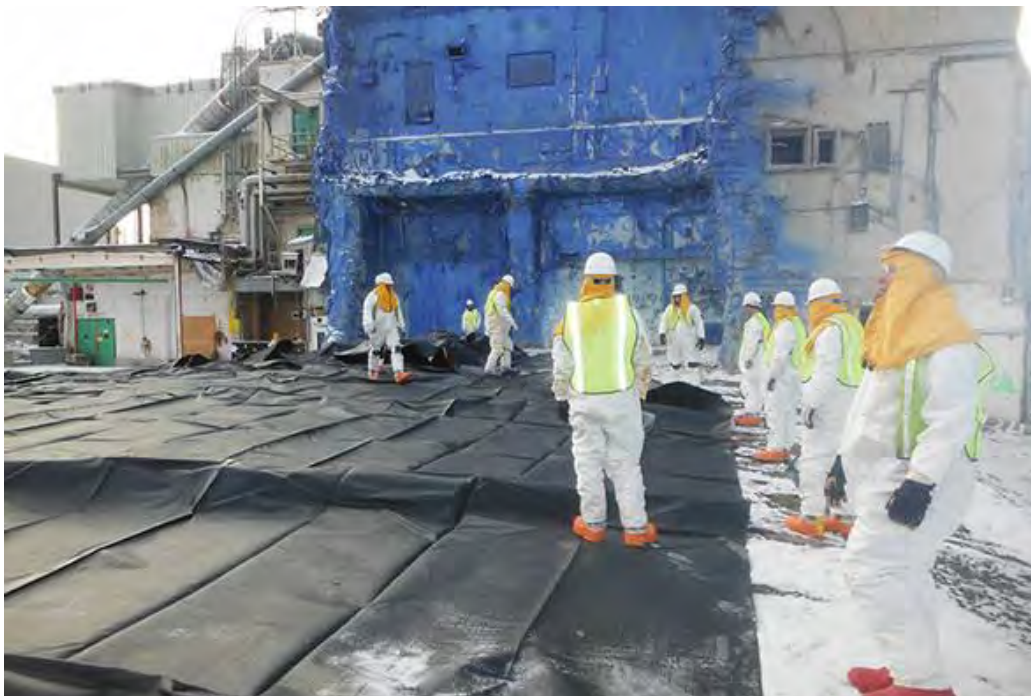
Workers pull and smooth out the cover over the Vitrification Facility concrete slab. The Main Plant, which is in the process of being deactivated, is in the background.
