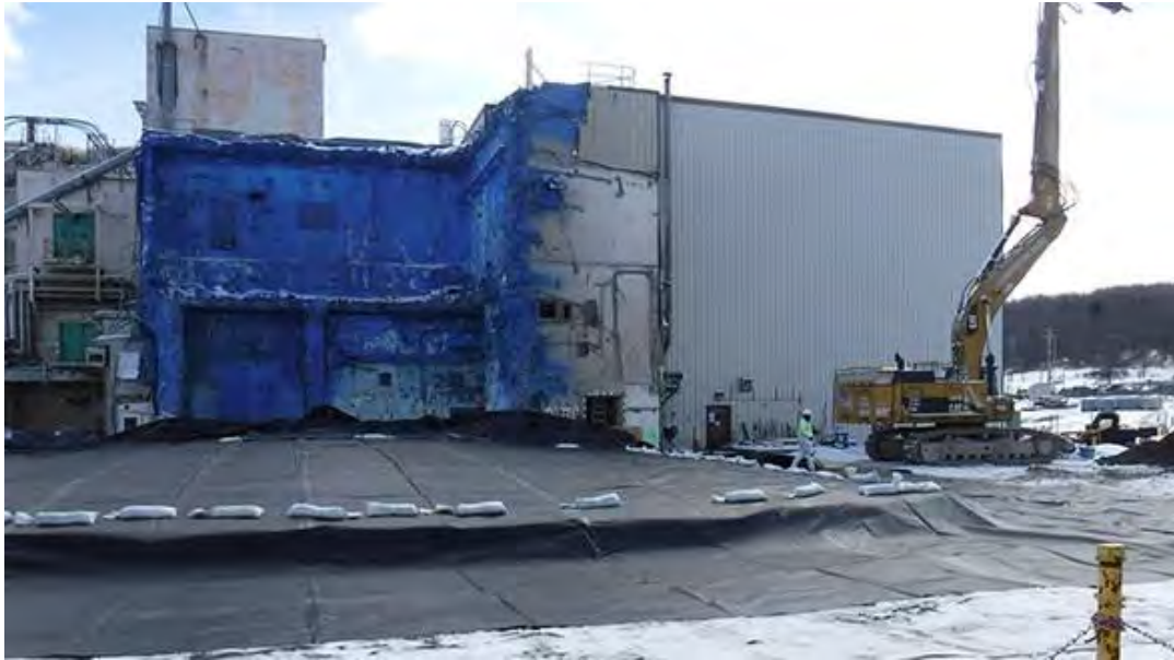
The Vitrification Facility demolition area after installation of the cover. The Main Plant, which is in the process of being deactivated, is in the background.
