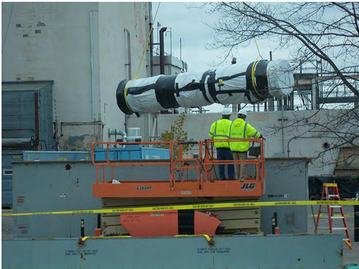
*CH2M HILL BWXT West Valley workers remove a 900-pound section of the ventilation exhaust cell duct from the roof of the Main Plant Process Building in November 2018.*
