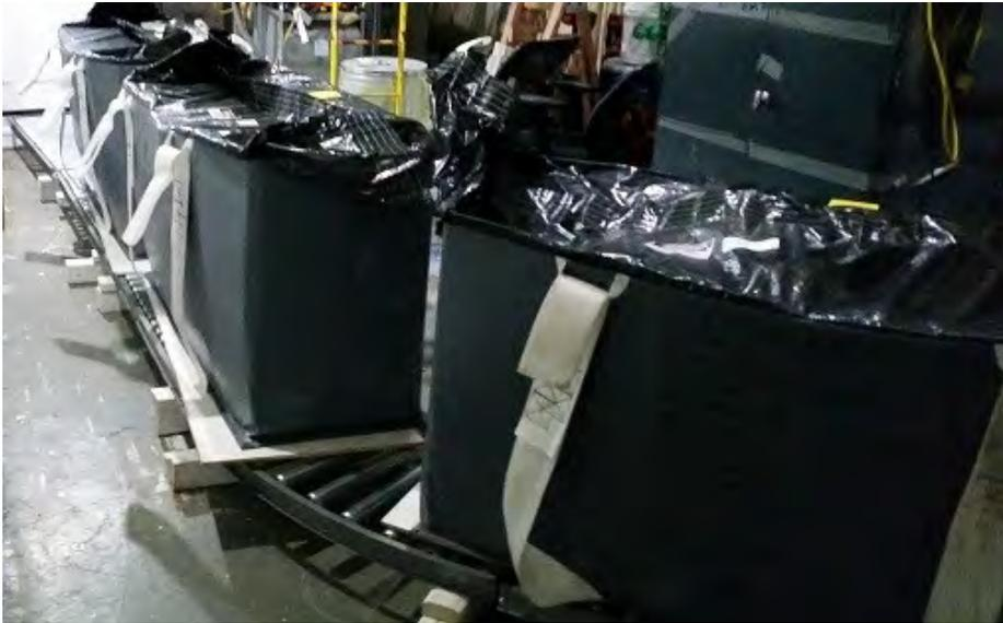
*Three 900-pound lift bags filled with asbestos material sit on a conveyor system designed by workers at EM's West Valley Demonstration Project.*
