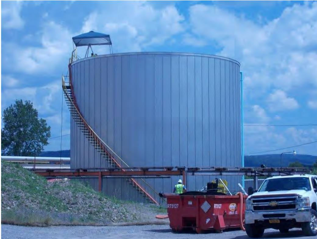
*EM conducts inspections of a 40-foot-tall fire storage tank at the West Valley Demonstration Project in accordance with National Fire Protection Association requirements.*
