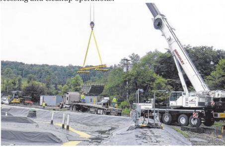
A crew offloads a section of interlocking concrete blocks called "armoring" that was used on the site's closed nuclear storage area to prevent soil erosion.
