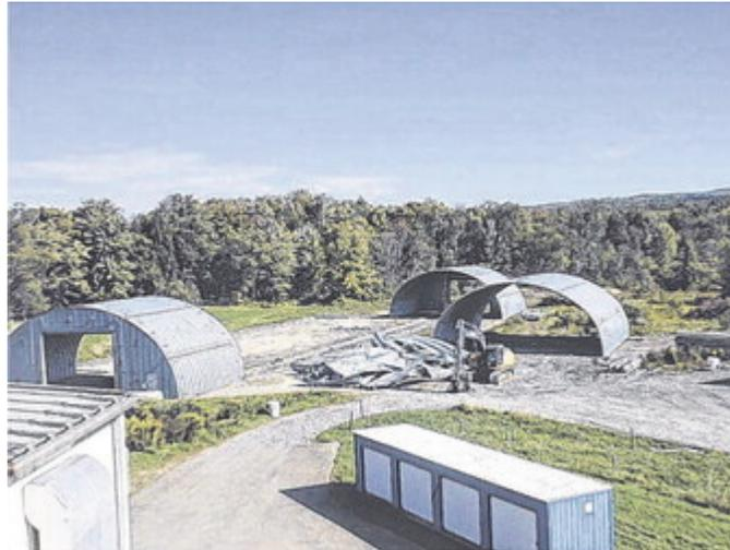
**An excavator with a shear attachment is used to demolish and size-reduce each section of the building. Debris was loaded into waste containers and shipped offsite for disposal.**
