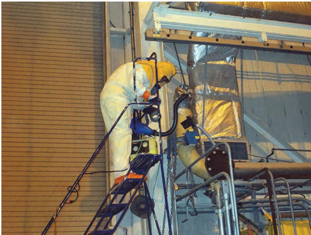
An operator inside the former fuel receiving and storage facility at the [West Valley Demonstration Project Site](#) pumps a fogging agent inside a pipe to fix suspected contamination. This work was part of deactivating the building for eventual demolition.
