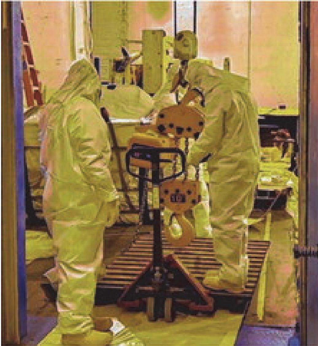
**Workers install a new hoist in the Equipment Decontamination that will be used for moving waste boxes and drums when the site returns to full operations; and crews resume deactivation work inside a former reprocessing cell there.**
