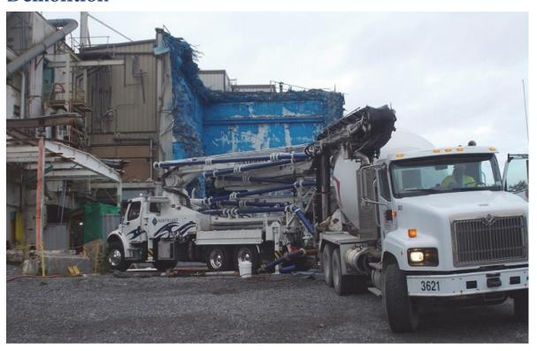
One of 44 trucks delivers grout to the West Valley Demonstration Project to place inside a cell 30 feet below ground.
