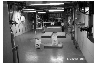
Cooling water pump removal, before (top photo) and after
