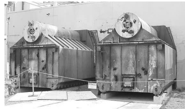
Boilers before and after stack removal
