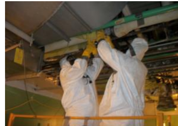
Asbestos abatement in Analytical Aisle
