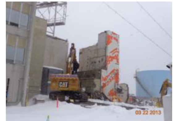
01-14 Demolition North Side Pipe Chase
