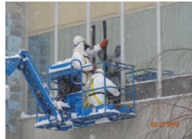
Window removal from MPPB Office
