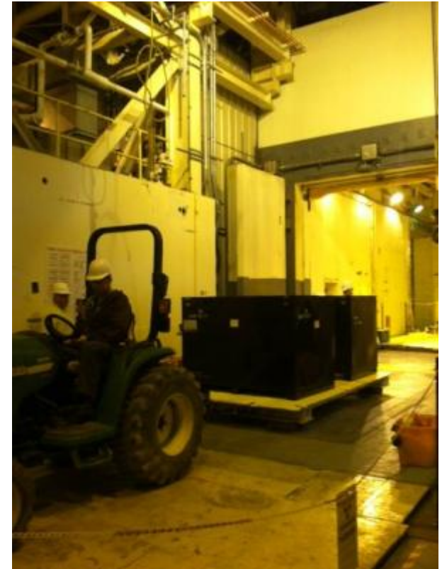
EDR Waste Removal for Shield Door Repair
