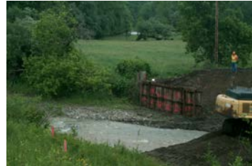
Bridge During Demolition Phase – June 10, 2013
