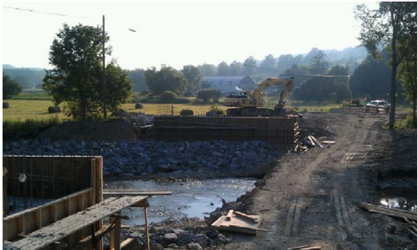
Bridge Construction as of 7-18-13
