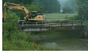
Bridge Just Prior to Demolition – June 6, 2013
