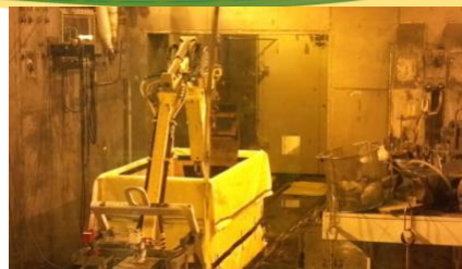
Downdraft Table Loadout in Vitrification Cell
