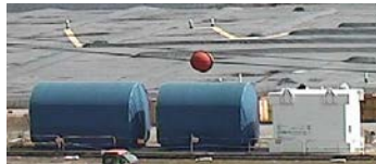
Vitrification Components will be Prepared for Shipment
