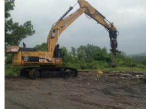
Piers Removal from WTF Test Tower Foundation
