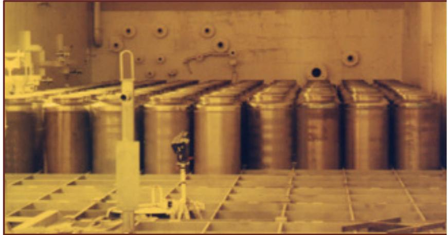
*Solidified high-level radioactive waste stored inside the Main Plant Process Building at the West Valley Demonstration Project is being relocated to prepare the structure for demolition. The multi-year relocation project involves building a storage pad and containers for the canisters, facility and equipment upgrades, and canister relocation.*
