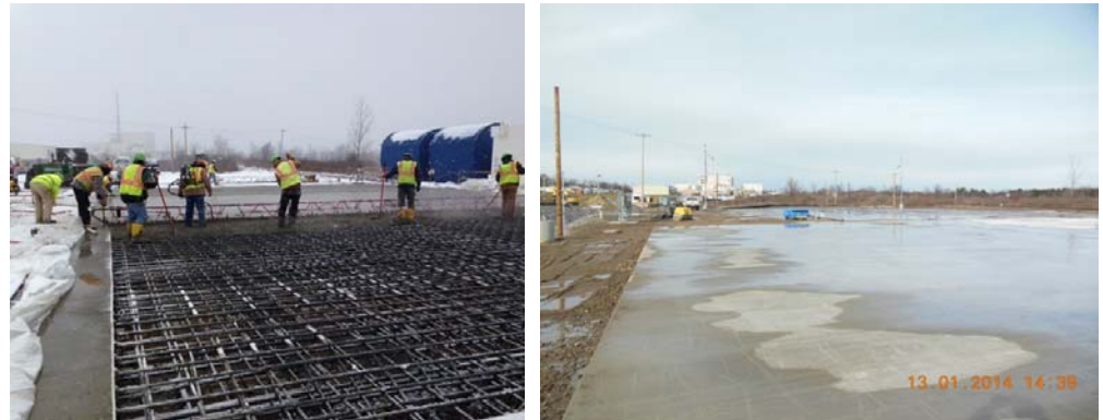
HLW Pad Construction and Completion
