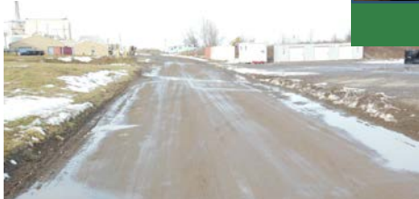
Haul Road Upgrades from MPPB to Storage Pad Planned for September/October
