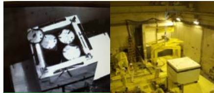
Remote TRU Drum Removal From HLWISF
