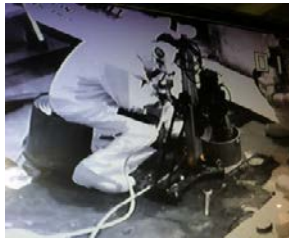
Core Boring in the EDR
