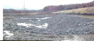
Construction Area Silt Fence
