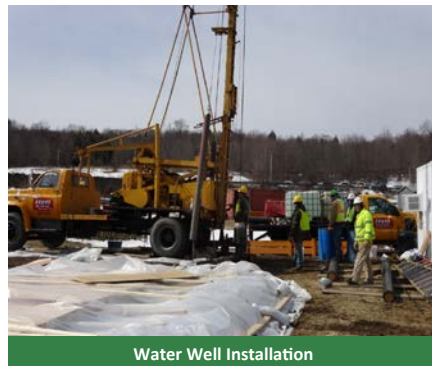
Water Well Installation
