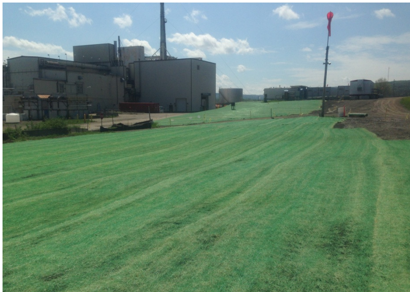
Restoration After Seeding and Mulching
