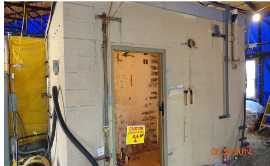
Con-Ed Building After Piping Removal
