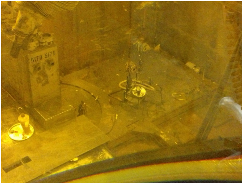
Vit Cell Equipment Pit West Side Vacuuming
