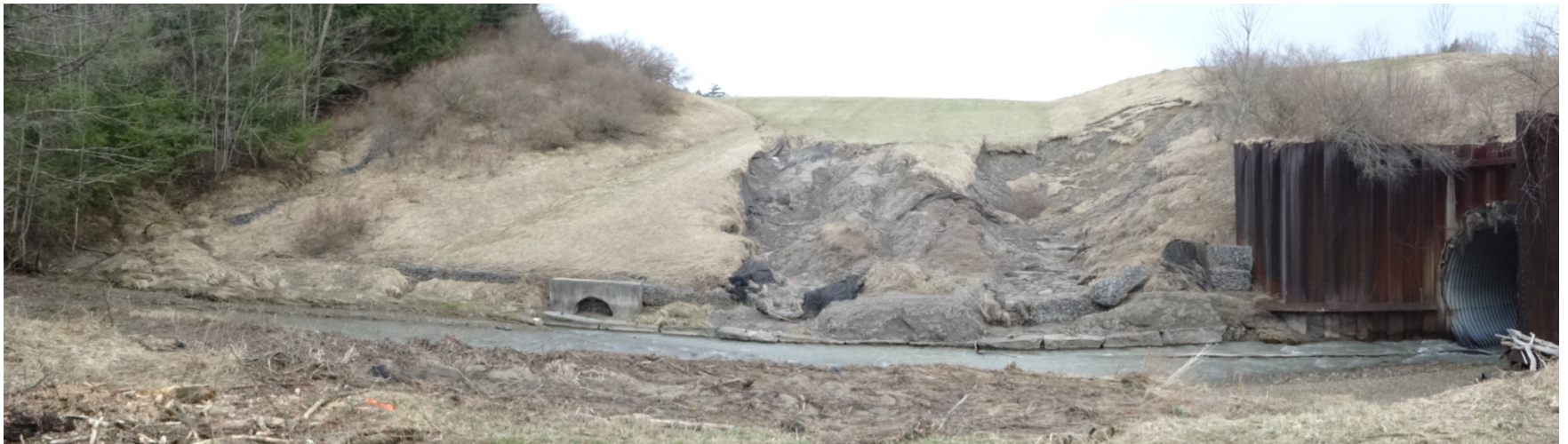
Documenting Weekly Inspection Lake 1 Spillway
