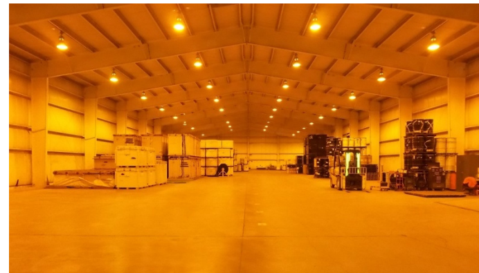
Lag Storage Facility Before and After 2013 Shipping Campaign
