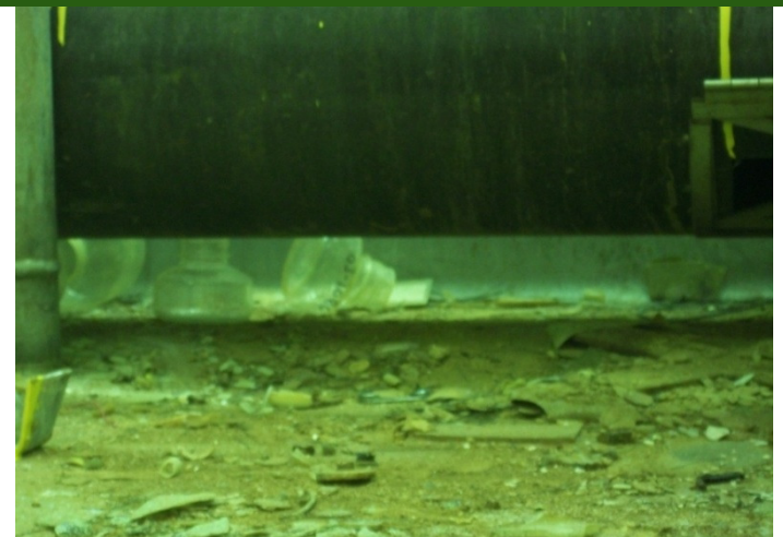
Analytical Hot Cell #4 Floor Conditions
