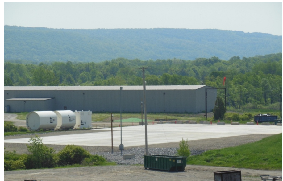
Completed Storage Pad
