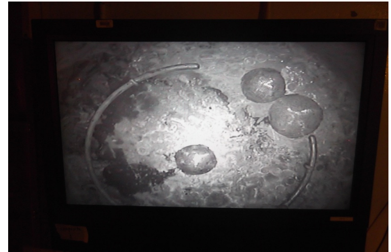
Bottom of Tank 13D-8 after Ring Removal
