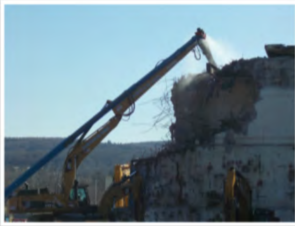
Removal of Vitrification Facility roof steel beam April 23, 2018
