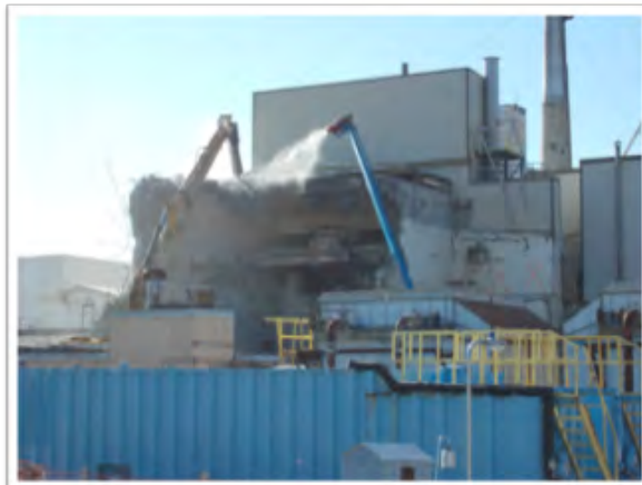
Demolition of Vitrification Facility roof April 23, 2018
