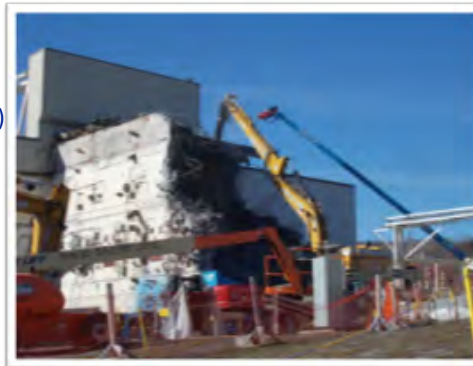
Vitrification Facility roof demolition April 23, 2018
