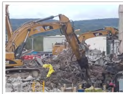
Vitrification Facility Demolition
