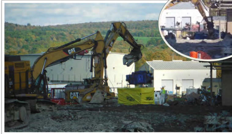
Contact Size Reduction Facility's dust collector being loaded during demolition
