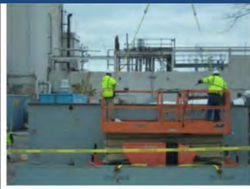
Removing VEC 36-inch duct from MPPB roof
