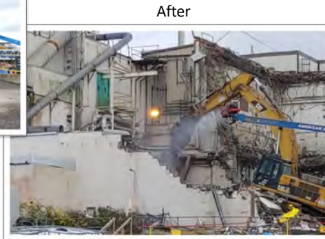
MSM Shop demolition
