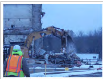
Waste disposition in Vitrification Facility demolition area
