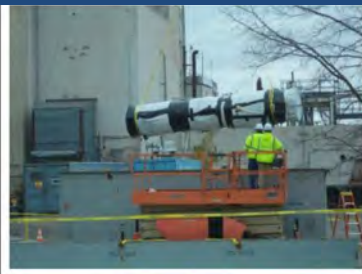
Removing VEC 36-inch duct from MPPB roof
