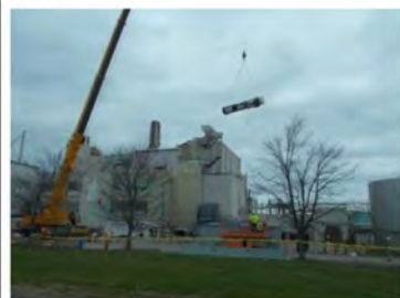
Removing VEC 36-inch duct from MPPB roof
