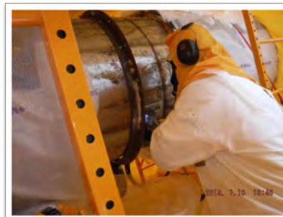
36-inch VEC vertical duct cutting
