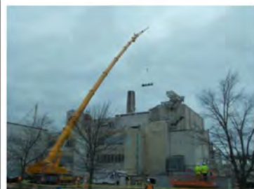
Removing VEC 36-inch duct from MPPB roof
