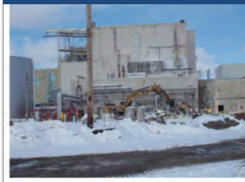
Demolition of Demineralizer Tank , Clarifier Tank and Connex trailer removal
