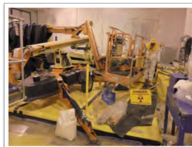
Inside Equipment Decontamination Room
