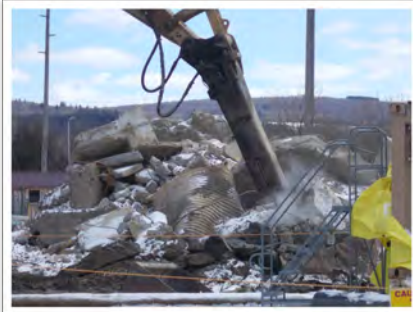
An excavator with hydraulic hammer is used to size-reduce concrete from the demolition of the Low-Level Wastewater Treatment Facility 02 Pad
