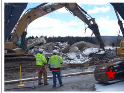
An excavator with hydraulic hammer is used to size-reduce concrete from the demolition of the Low-Level Wastewater Treatment Facility 02 Pad
