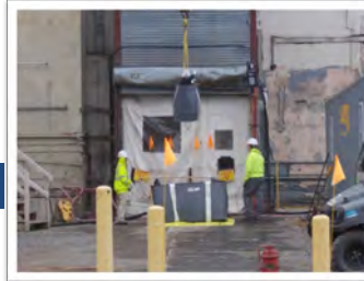
ACM removal from the fourth floor of the Main Plant
