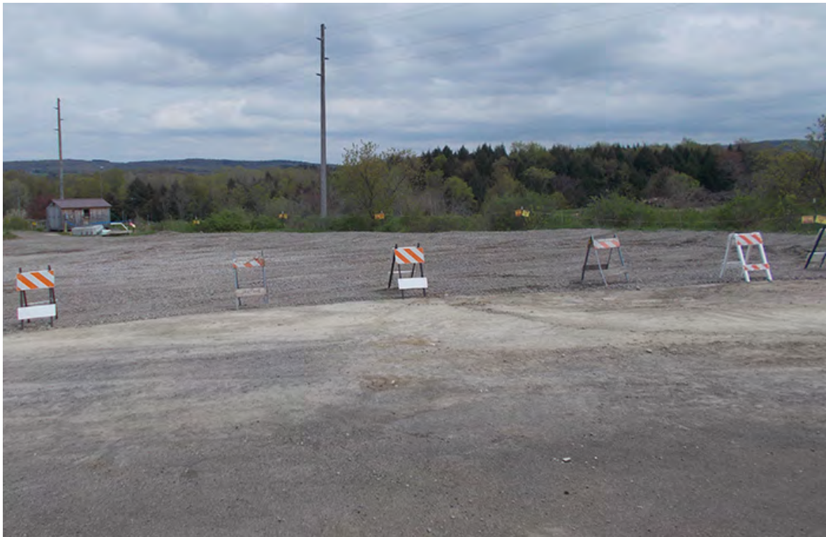
Workers recently completed the building pad demolition and restored the area.
