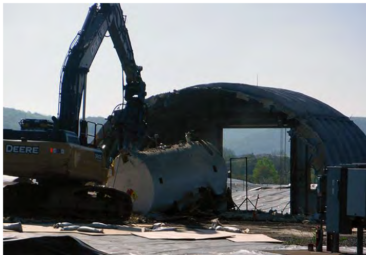
A crew tears down the liquid pretreatment system structure.
