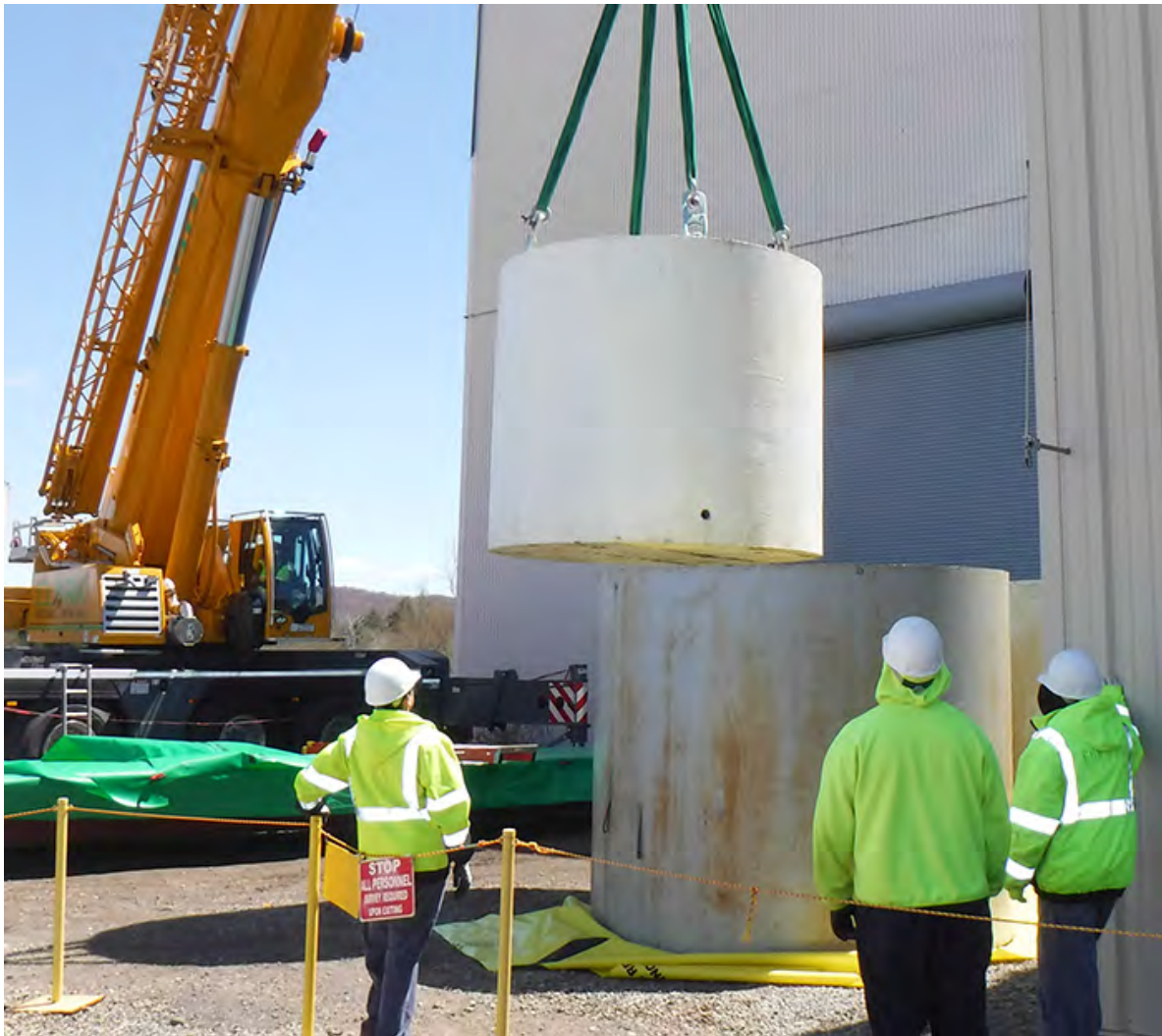
Using a 200-ton crane, workers return a waste container to its exterior steel shield at its new location at an outdoor storage area.
