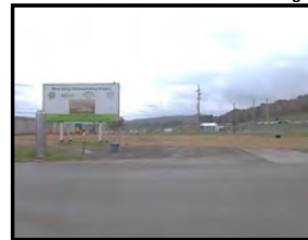
Demolition of Administration Building
