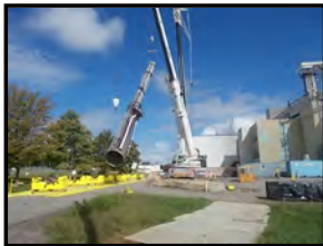
Removal of Upper Portion of MPPB Stack
