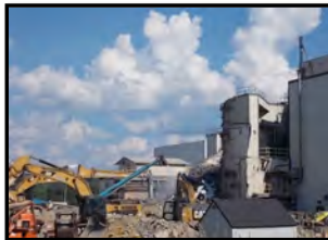
Demolition of Vitrification Facility
