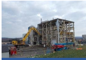
Load-In Facility demolition
