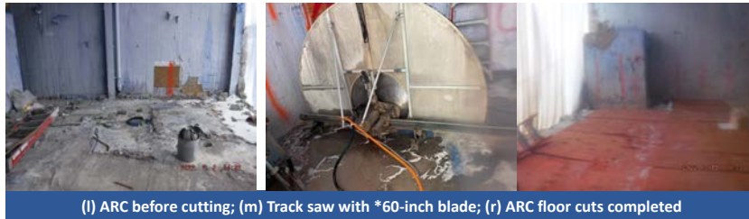
(l) ARC before cutting; (m) Track saw with *60-inch blade; (r) ARC floor cuts completed
