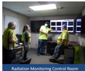
Radiation Monitoring Control Room
