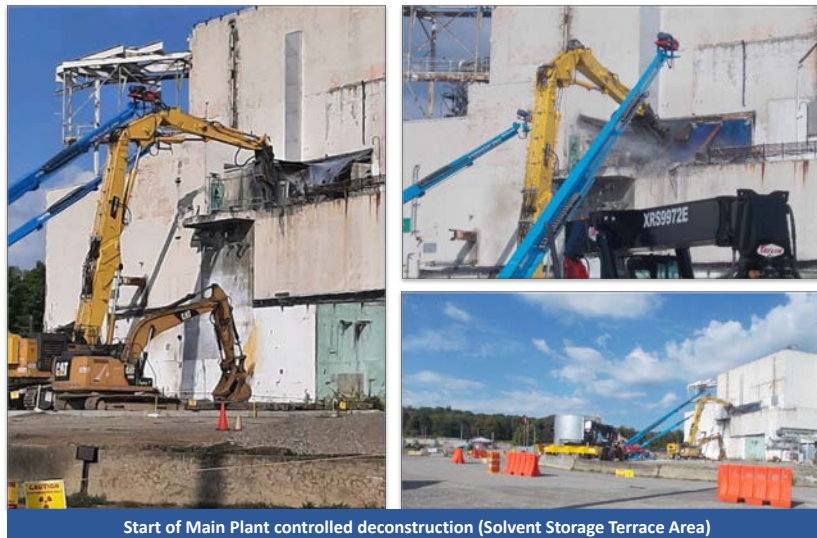
Start of Main Plant controlled deconstruction (Solvent Storage Terrace Area)
