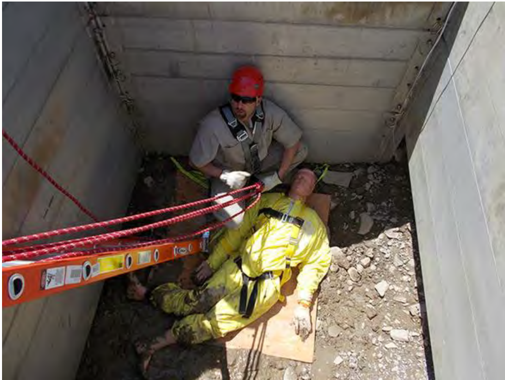
Eric Fuller of CH2M HILL BWXT West Valley takes his turn rescuing a 185-pound mannequin from the excavation pit during confined space training.
