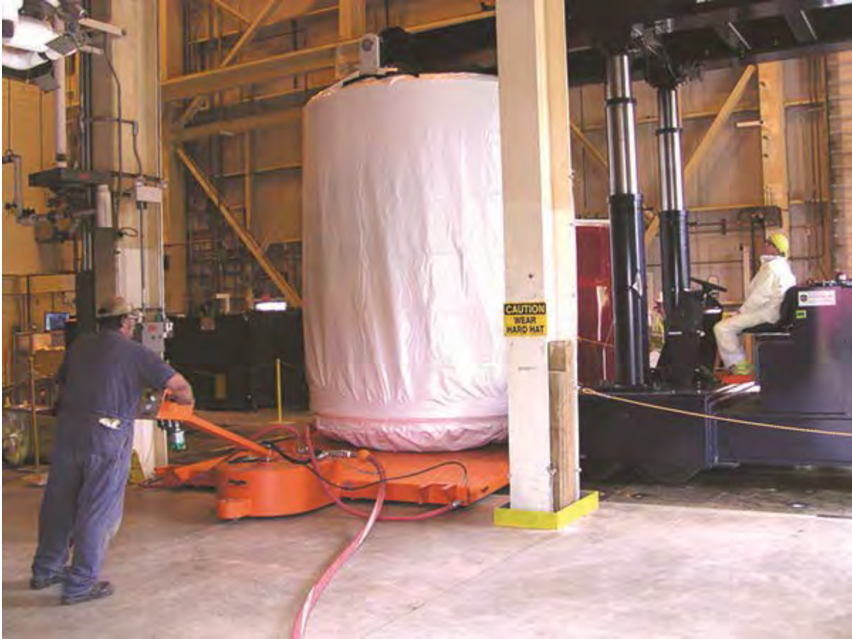
2. Safe cask transport in tight clearance. Courtesy: AeroGo Inc.
