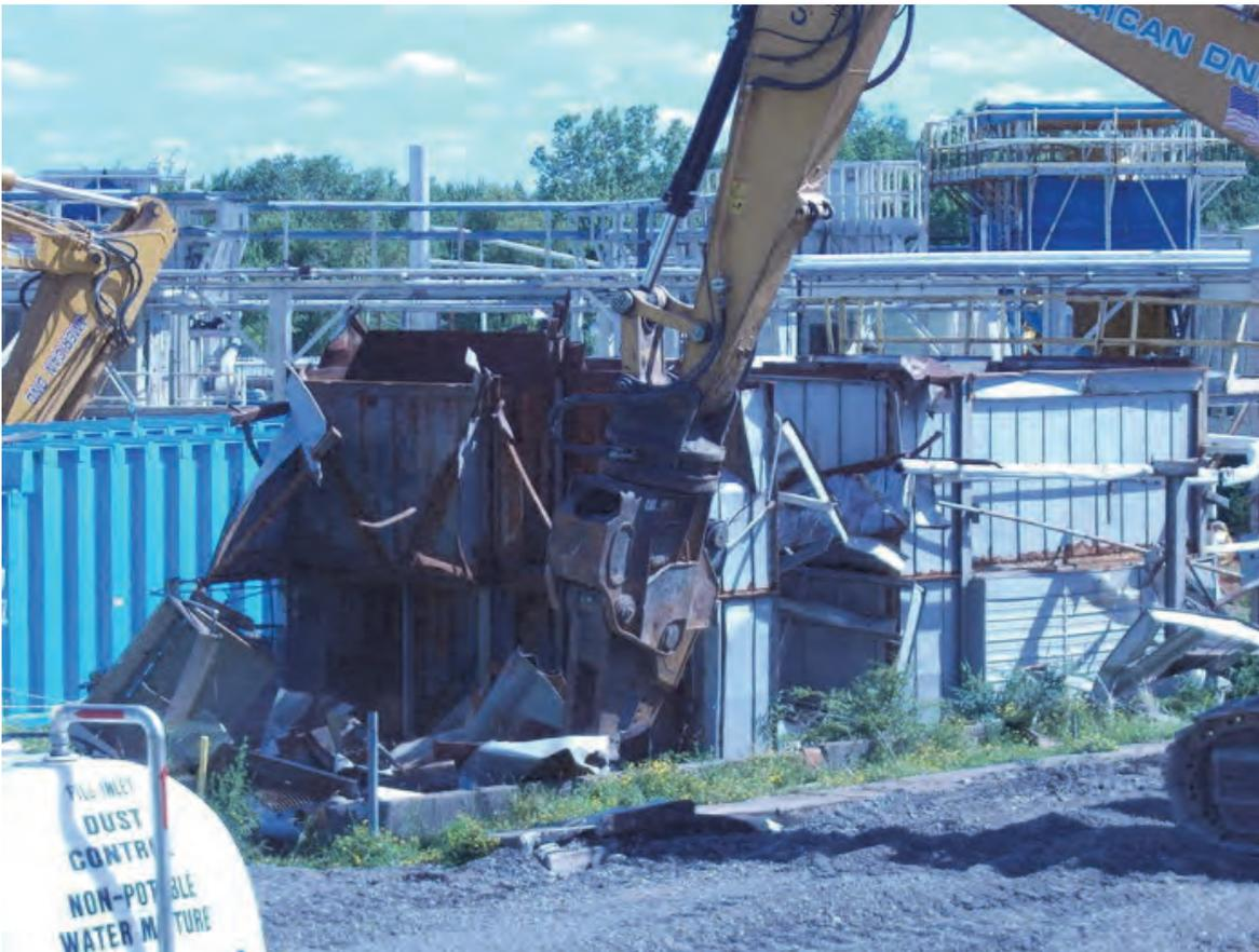
*An operator uses a hydraulic shear to remove one of two Waste Tank Farm condenser structures at the West Valley Demonstration Project.*
