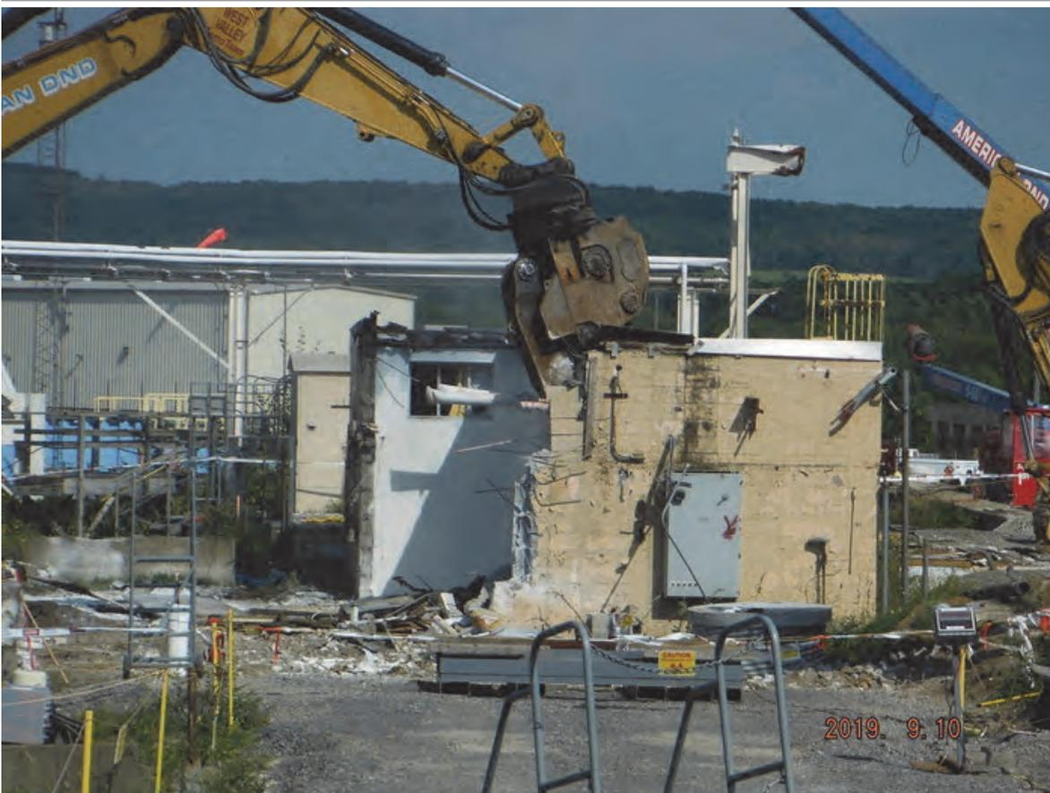
*An operator begins demolishing the Waste Tank Farm Shelter after completing the removal of two condenser structures.*
