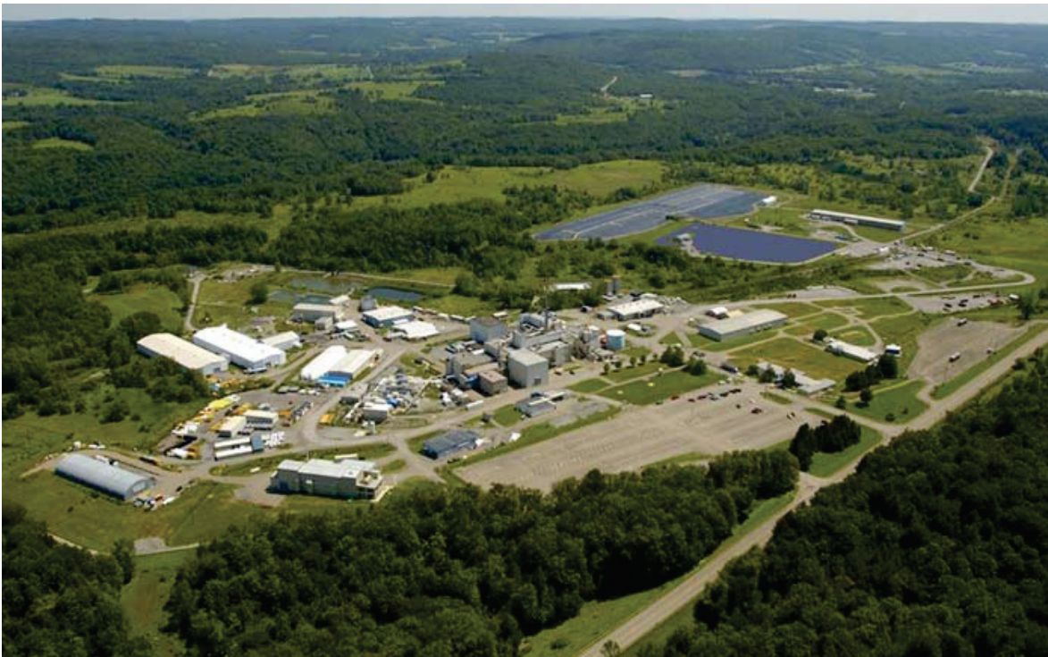
An aerial view of the West Valley Demonstration Project Site.
