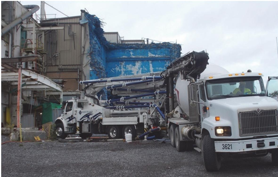
One of 44 trucks delivers grout to the West Valley Demonstration Project to place inside a cell 30 feet below ground.
