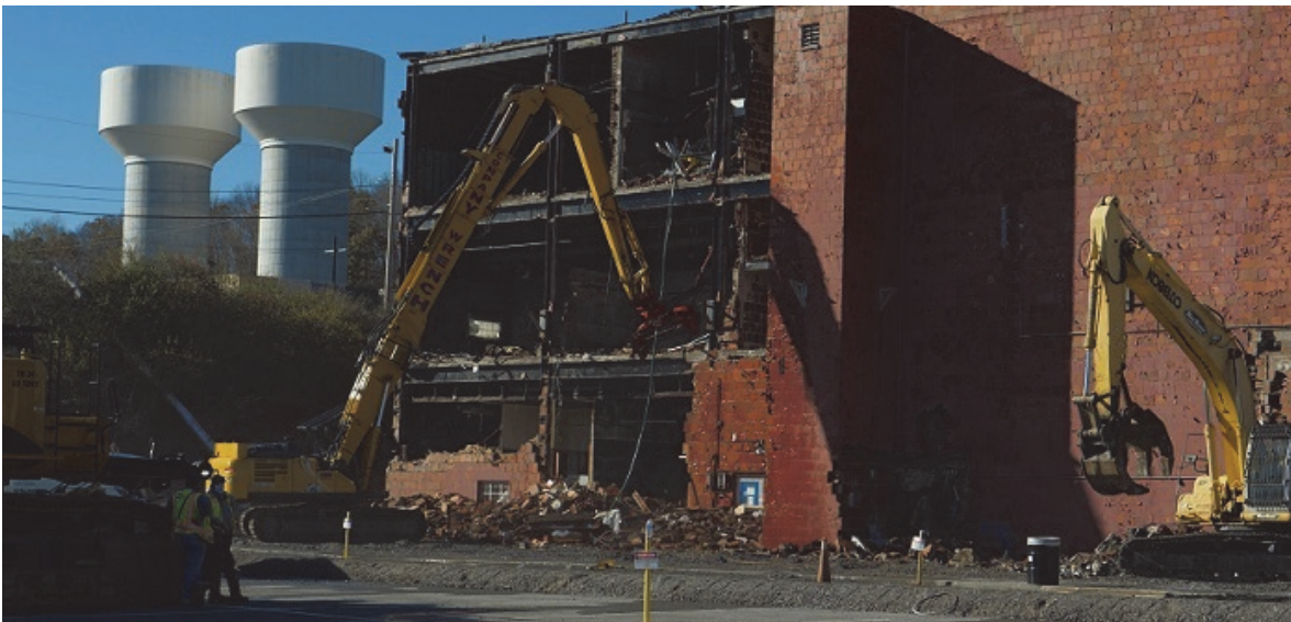
Crews demolish Building 9210 at the 1940s-era Biology Complex at Oak Ridge.
