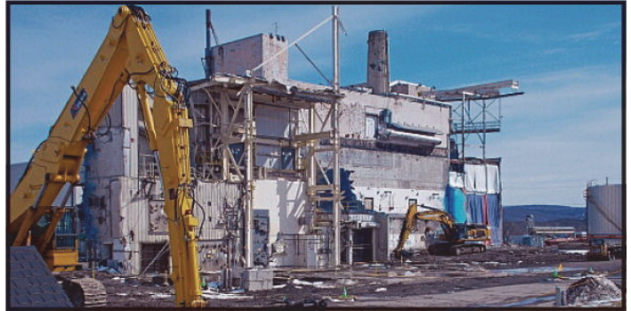
Workers complete the demolition of the Load-In Facility (March 2022)
