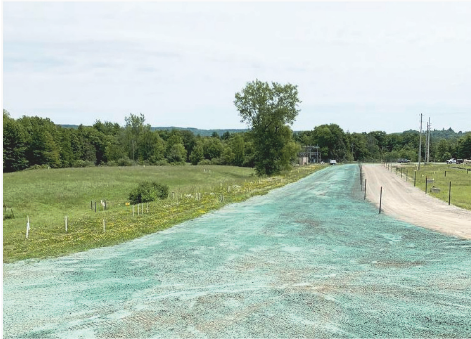
The permeable treatment wall soil and structure project area is restored with hydroseed, a technique that spreads a specialized, semiliquid grass mixture evenly over bare ground to grow grass and prevent soil erosion.
