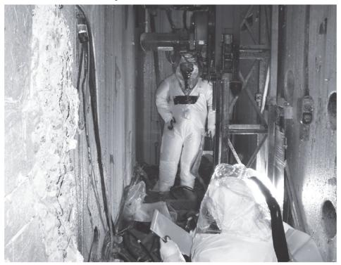
Photo provided Workers completed the deactivation of the Product Purification Cell-South and have applied fixative for contamination control as part of the deactivation process. The cell had previously contained high levels of contamination from former fuel reprocessing operations.
